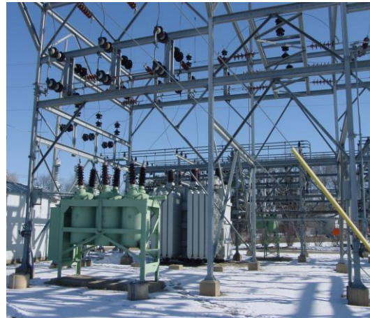
Pheasant Branch Before Construction
