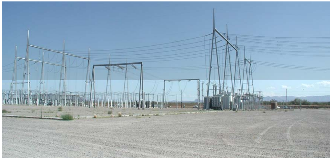
SAGUARO YARD PRIOR TO CONSTRUCTION 08/2002
