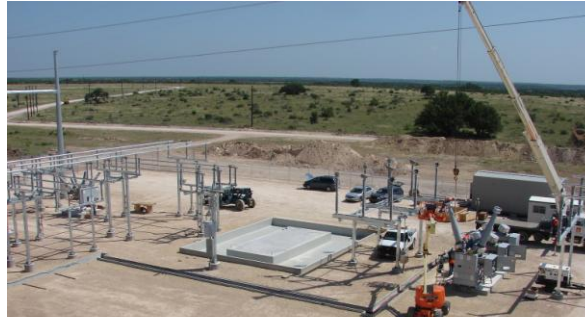
Site Under Construction
